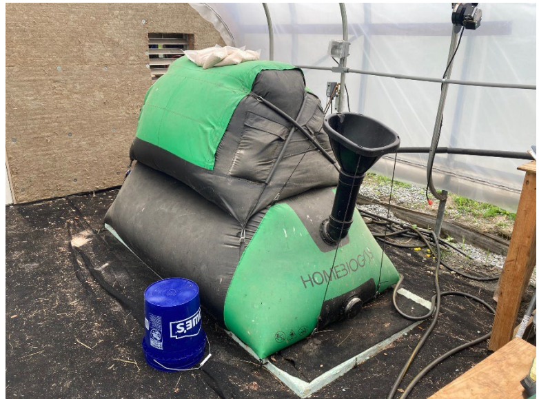
Our Home Biogas digester generated the effluent from food waste.
