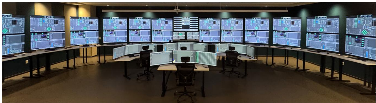
Figure 1. SMR Control Room Simulator used in the simulation-based clean-energy laboratory
