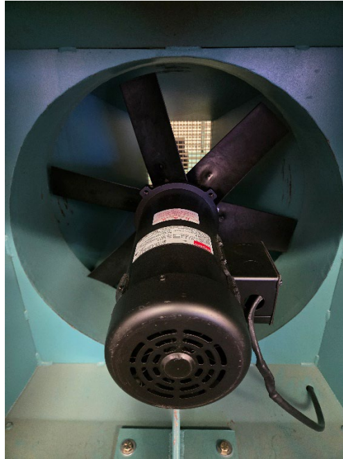
Figure 2: New Dayton DC permanent magnet motor and composite 6-bladed axial fan.
