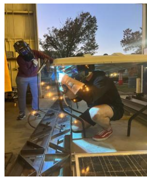
Figure 9: Process of Roof Reinforcing
