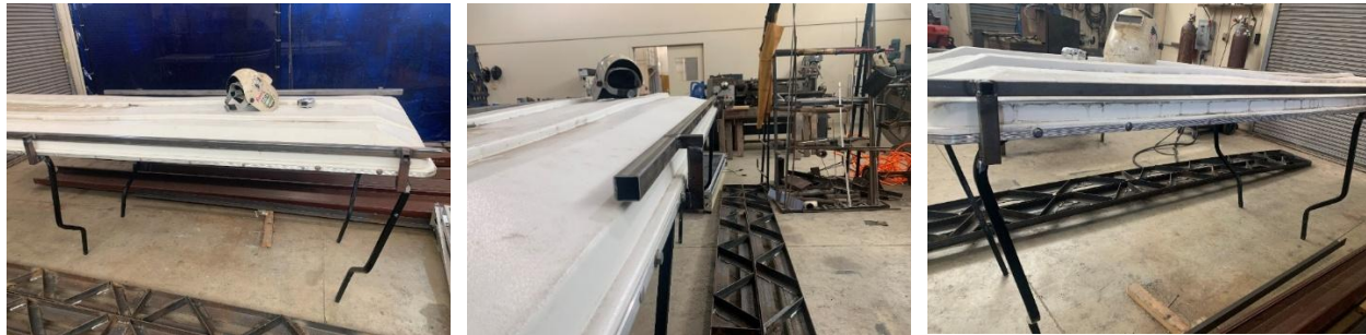
Figure 11 – a) A side view of the added bars. b) A front view of the welded bars. c) Side view of the bars.
