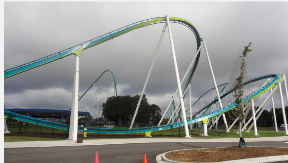
Figure 3: The roller coaster Fury 325, pictured here before a crack shut down operations. (‘Fury 325’ by Martin Lewison is licensed under CC BY-SA 2.0.)
