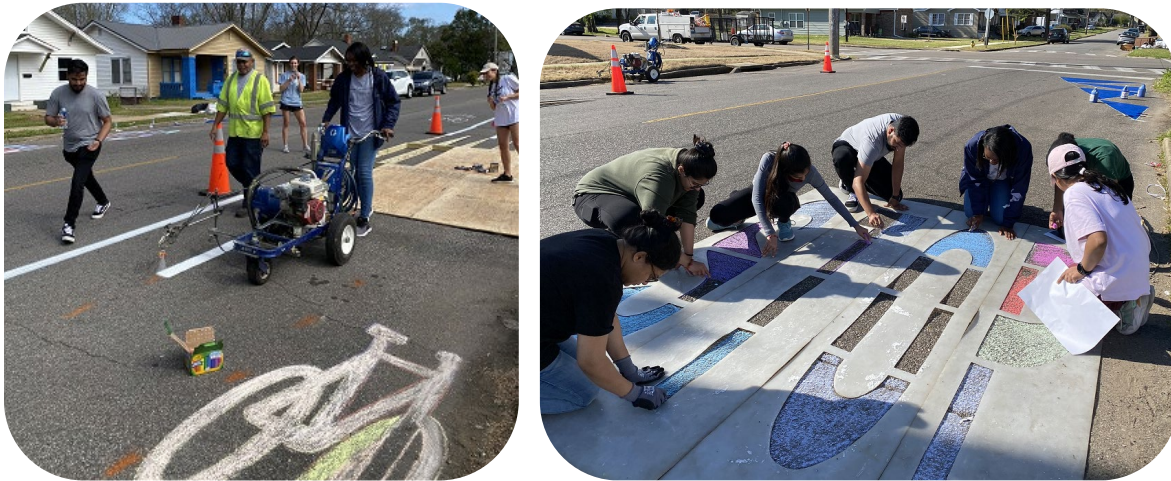
Figure 7. Students Installing a Traffic Calming Initiative, Painting a Bike Lane and a Bus Stop Bulb Out in Collaboration with the City of Birmingham Department of Transportation
