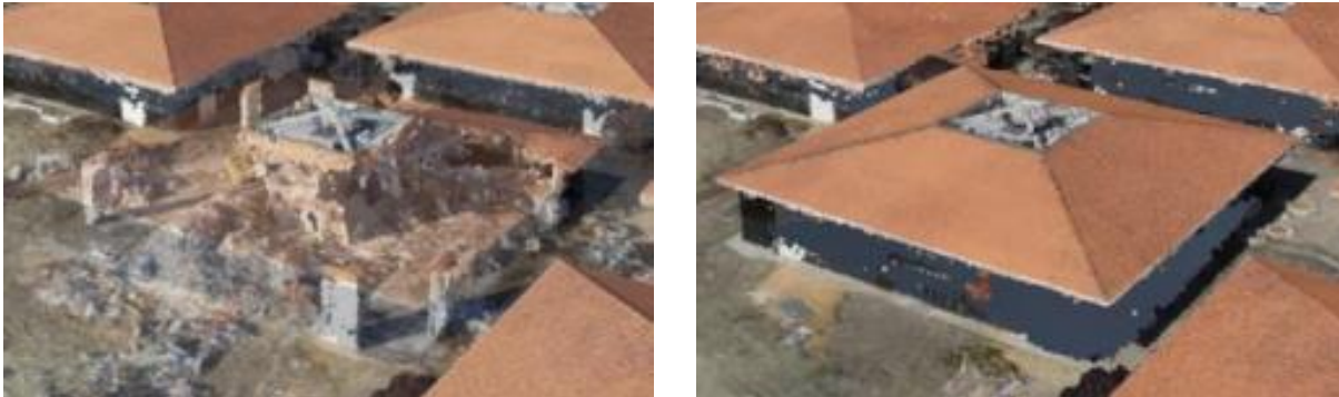
Figure 3 Example of construction progress in time-lapse [8]
