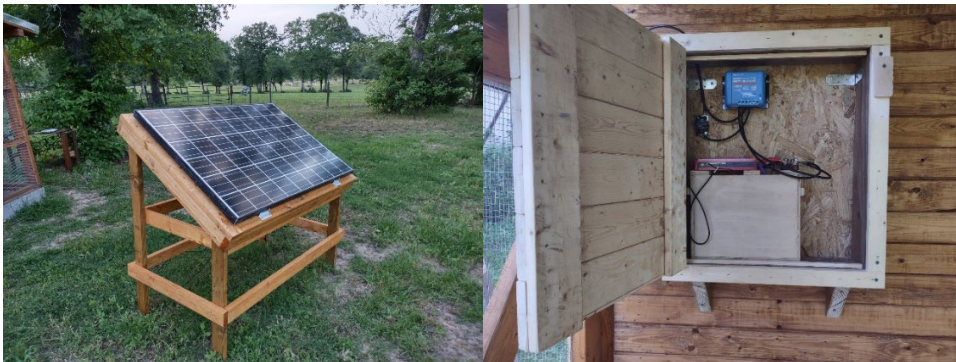
Figure 2. PV Panel Install and Charge Controller
