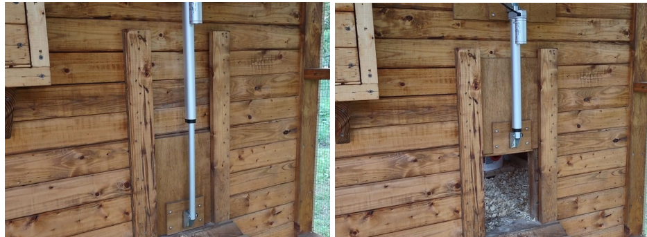
Figure 6. Automated Coop Door Closed and Open
