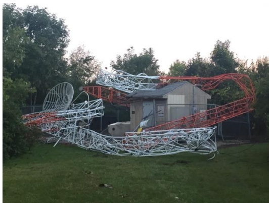
Figure 3: Radio tower in Galion, Ohio after the tornado
