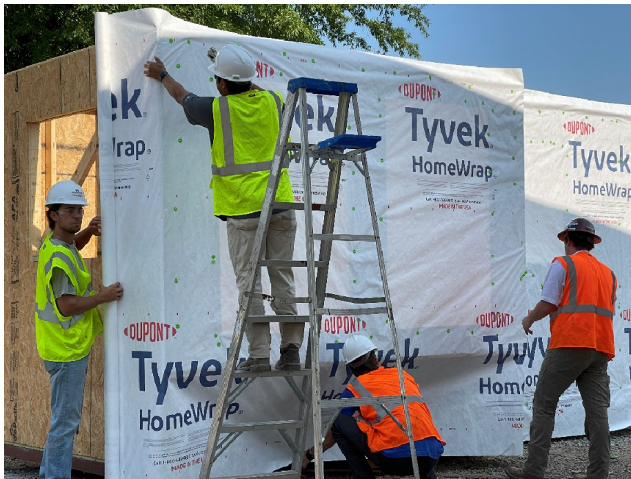
Figure 2. Students are working on completing the placement of the weather barrier on the building.
