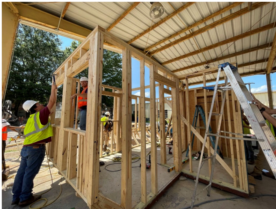
Figure 1. Students are working on completing the wood framing outside.
