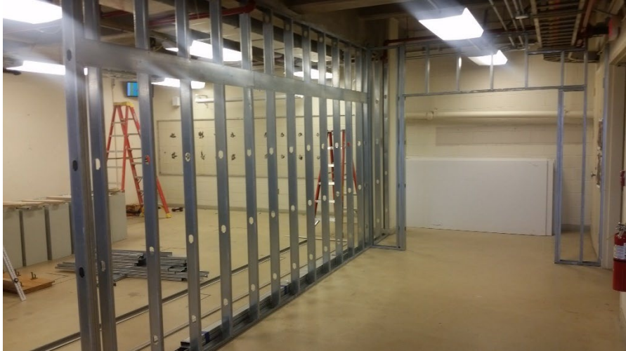
Figure 9. Soil Mechanics Classatory During Renovation
