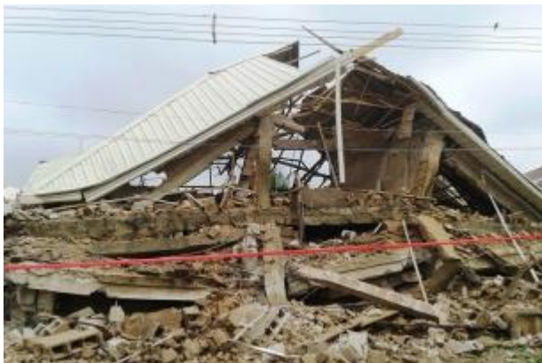
● A collapsed building [12]
