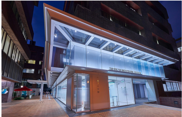
Figure 1a. Transparent design connects student innovation in engineering and technology with the public, establishing it as an iconic landmark on campus.
