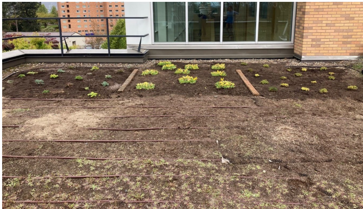
Figure 2. Planting on Green Roof during Year 1 (stone crop on the left, sedum mix in the middle, thyme on the right)
