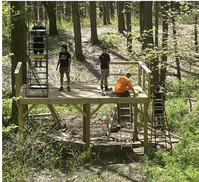
Figure 4. Finished zipline tower
