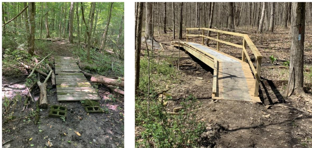
Figure 7. The Previously Existing Bridge and the New Bridge
