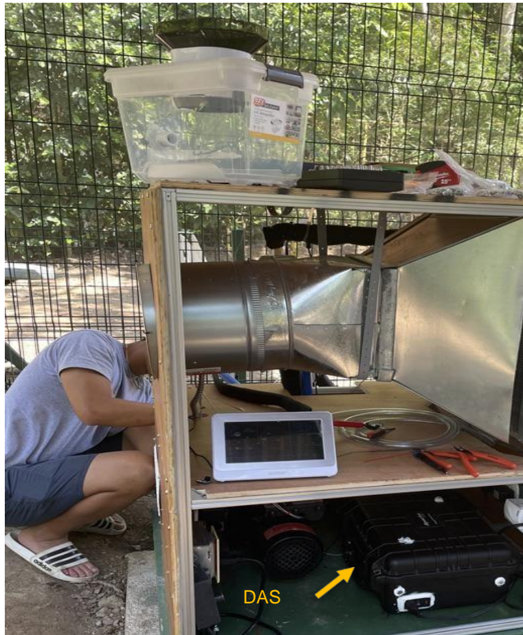
Figure 9: The figure above shows a photo of the final location of the DAS.
