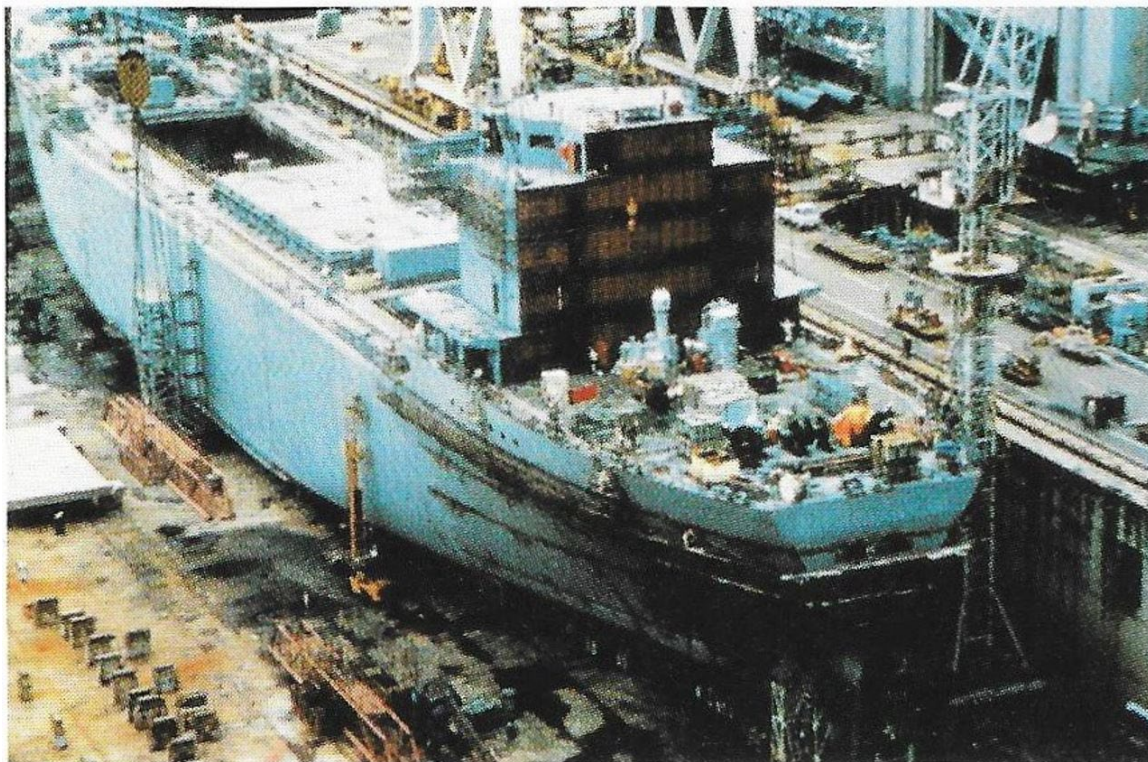
Figure 5 – Assemble of Forward Deckhouse Module (or Unit or Block) [12]
