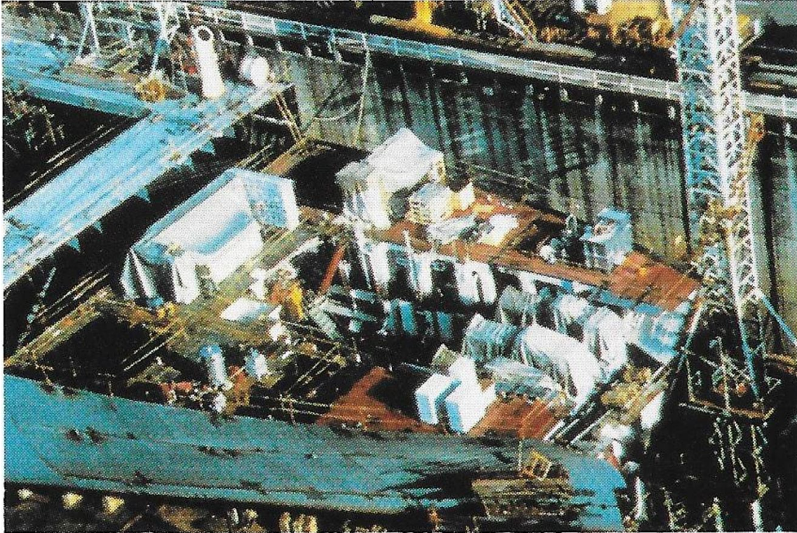
Figure 2 – Assembly of Machinery Modules (or Units or Blocks) [12]
