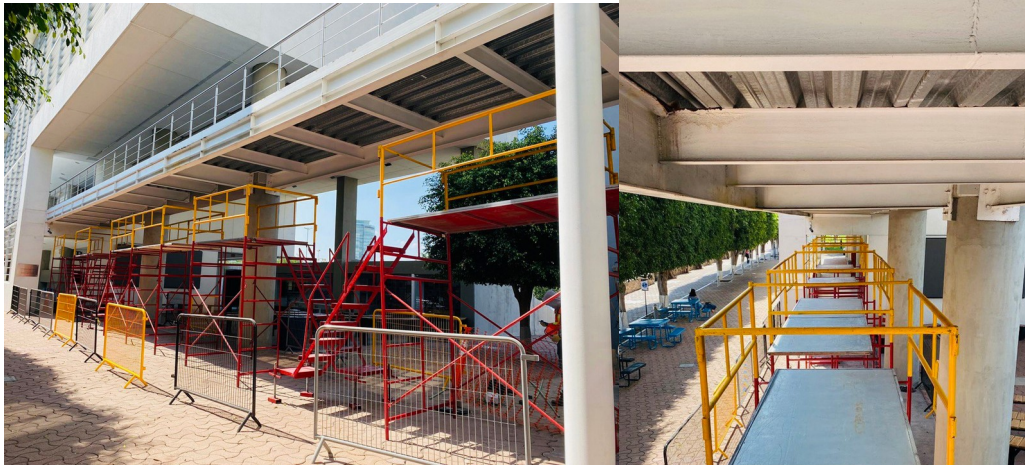
Fig. 5 Steel bridge in Campus BBBB.
