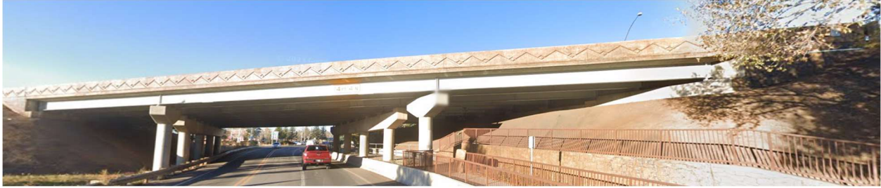
Figure 3: The McConnell Bridge carrying I-17 at the southwestern corner of NAU. [13]
