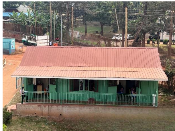
Figure 7: Exterior of Makerere DesignCube
