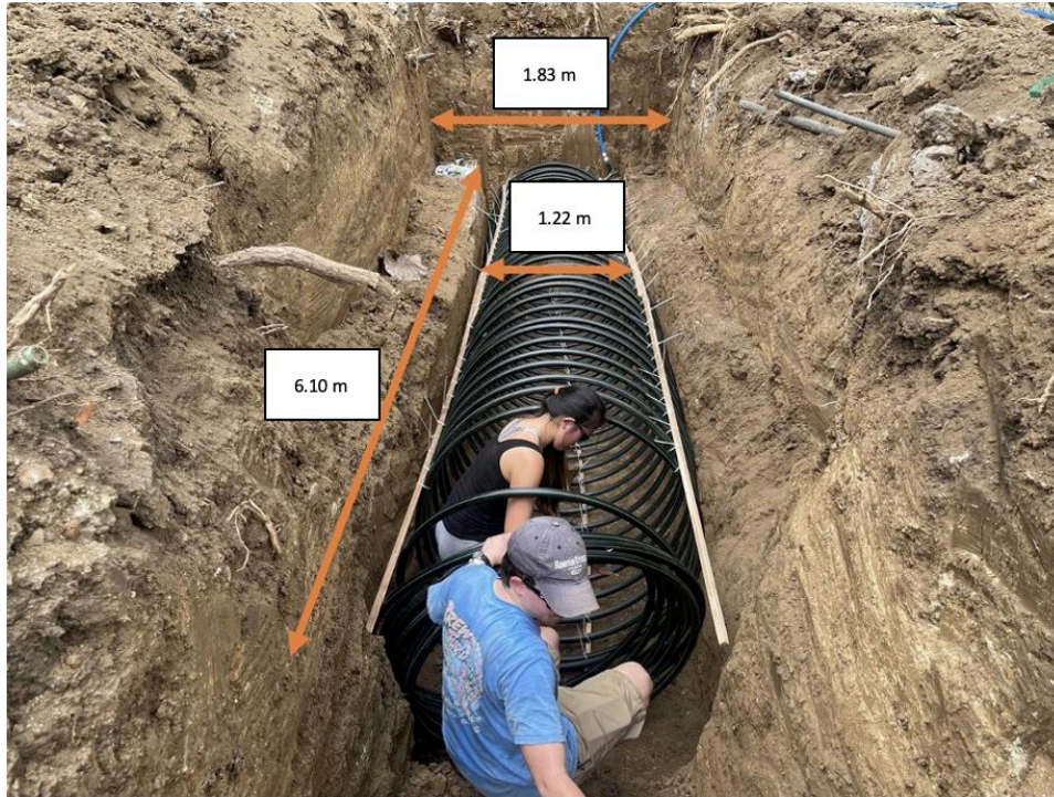
Figure 6: Installing the Underground Geothermal Piping
