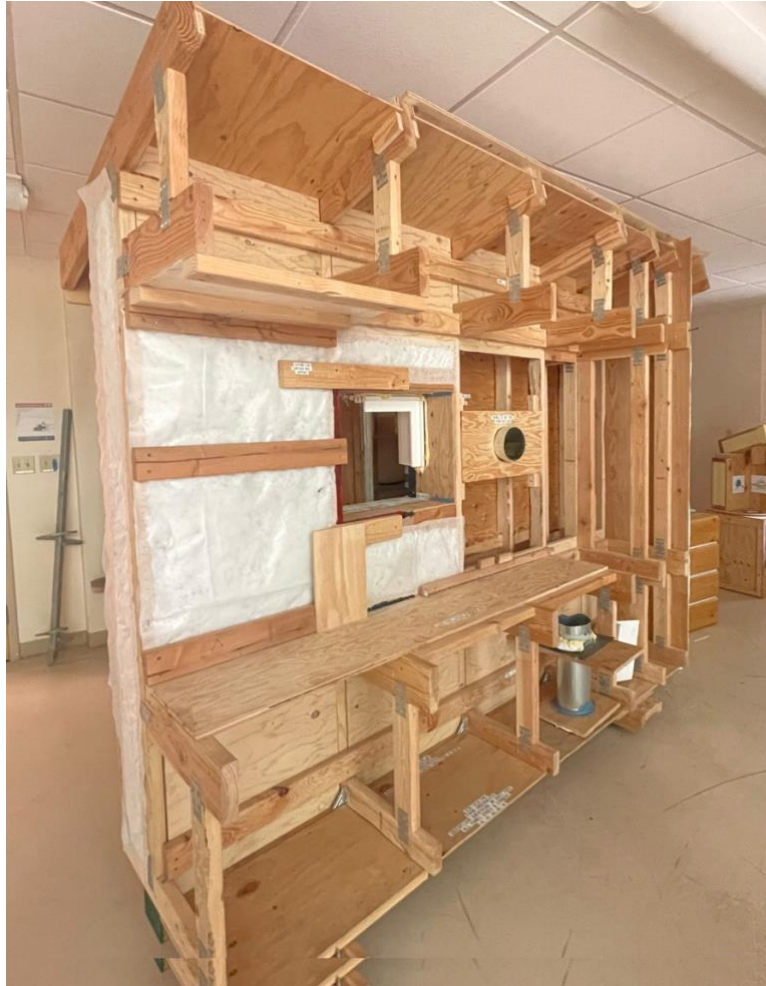
Figure 3. Full view of integrated truss demo. Photo by Todd Nicewonger, 2022.
