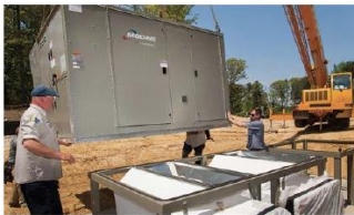
Picture Caption: HVAC system is being installed at a new facility
